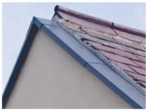
Sealant must be applied to the inside edge of the WEC 771 OVERTRIM.
